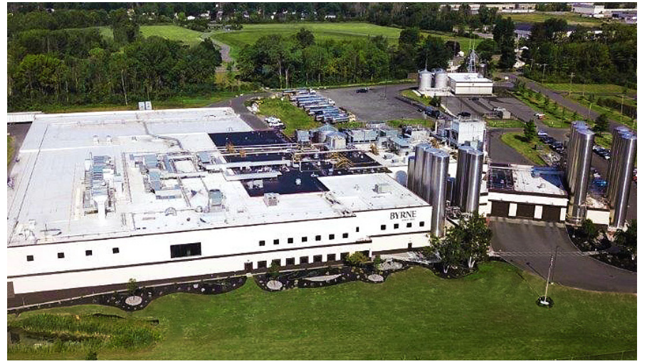
Byrne Dairy received a $1 million Northeast Dairy Business Innovation Center grant to purchase and install a new UHT processing system at the company's DeWitt facility, resulting in a 20 percent increase in the amount of milk processed.
